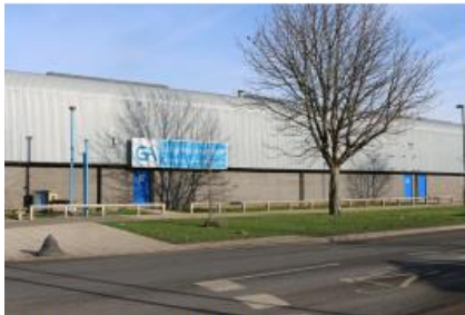
1 - Blank frontages on Surrey Canal Road
