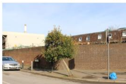
6 - Blank walls surrounding waste management
